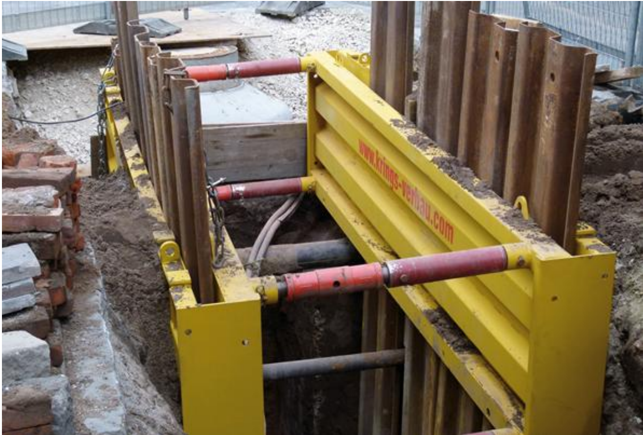
↑ Universal DKU piling frame element
