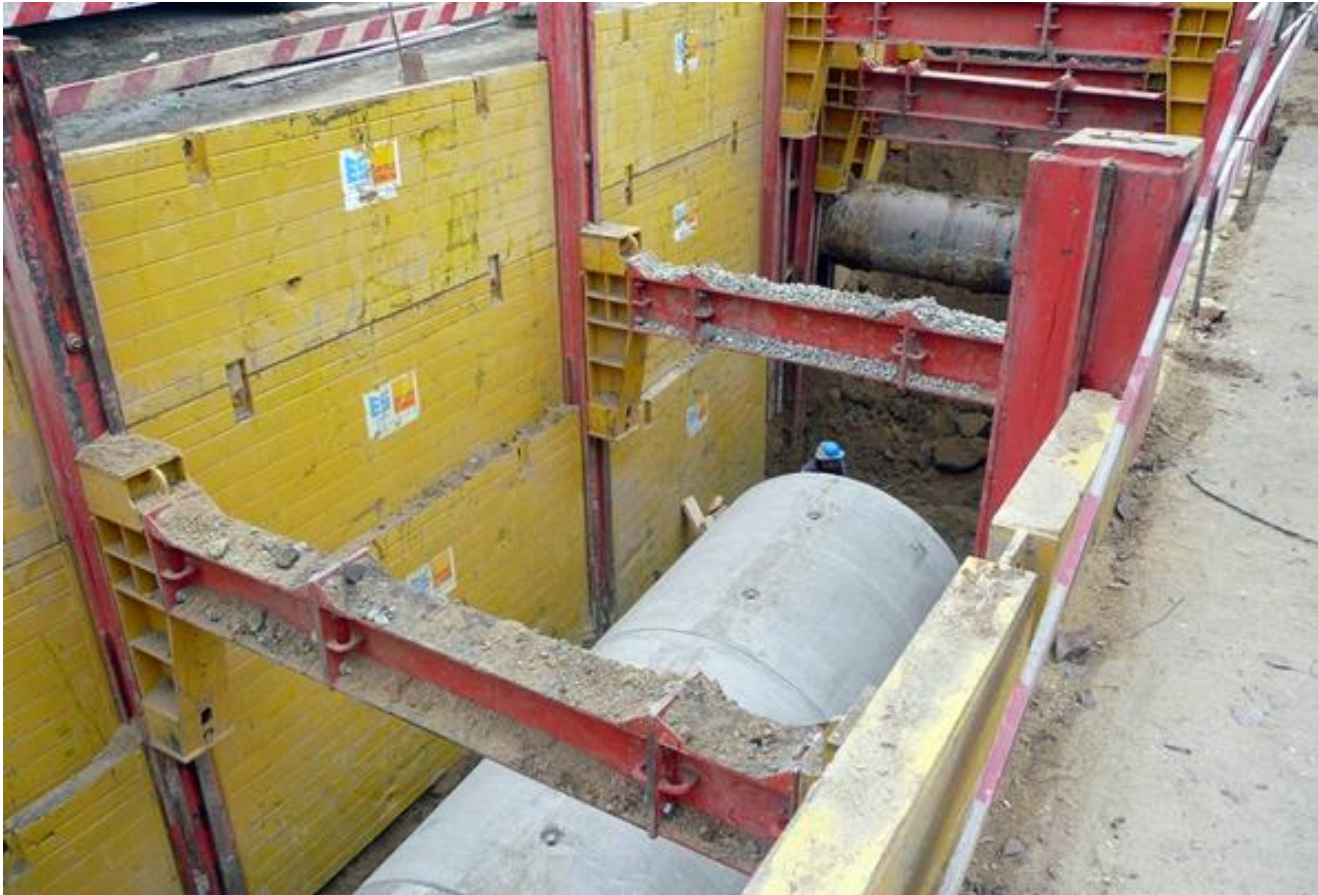
↑ Double slide rail system, parallel shoring, DG PV
