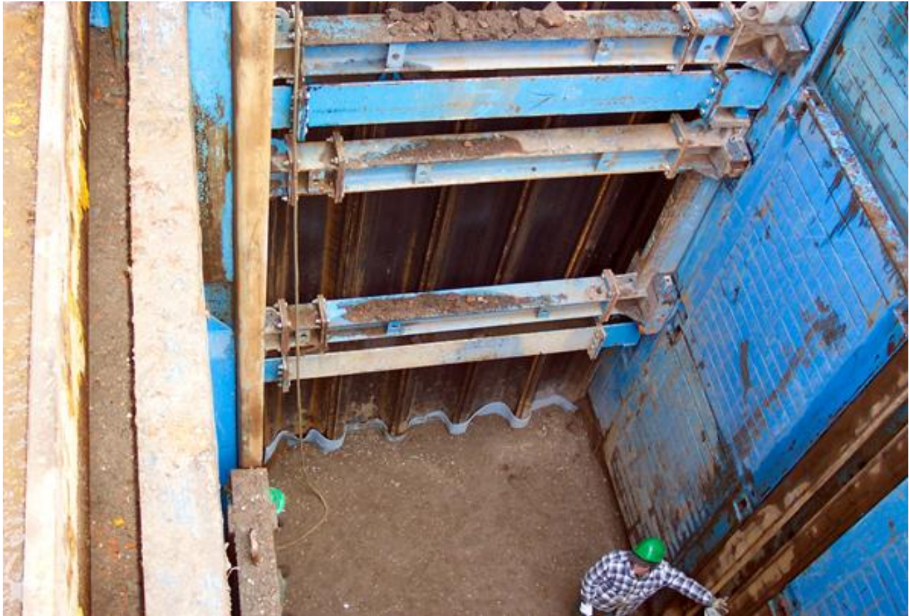
↑ Head shoring with sheet piles
