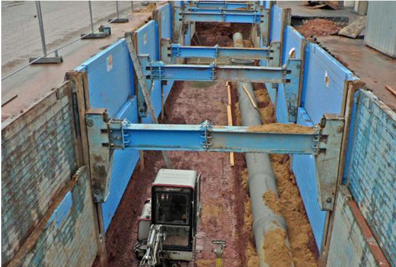
↑ Double slide rail system Linear shoring with U-type boogie car
