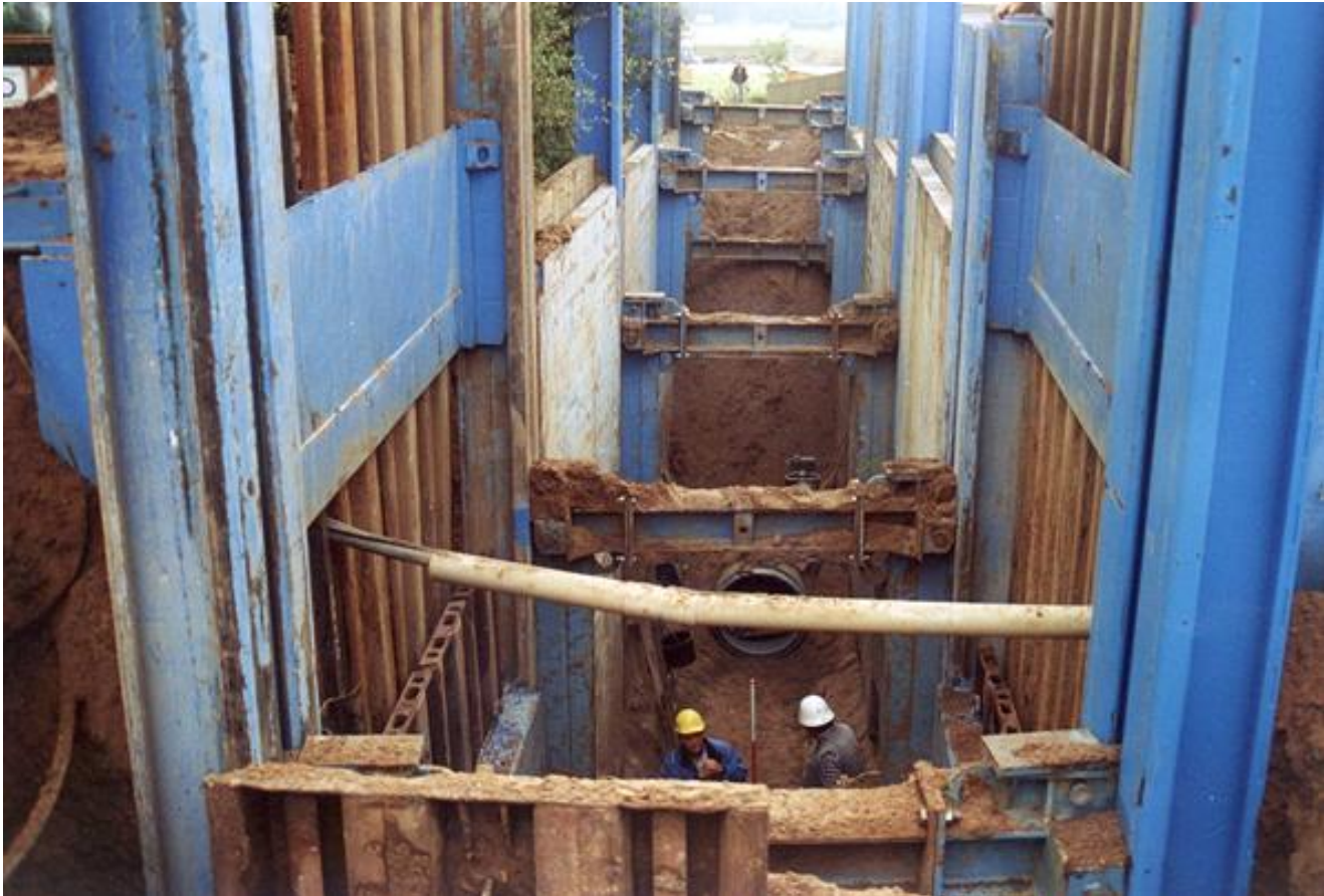
↑ Double slide rail innercity shoring
