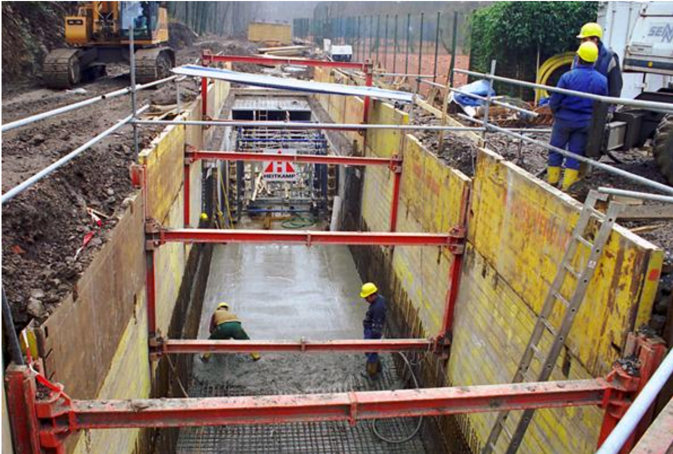
Single slide rail system, parallel shoring, EG PV
