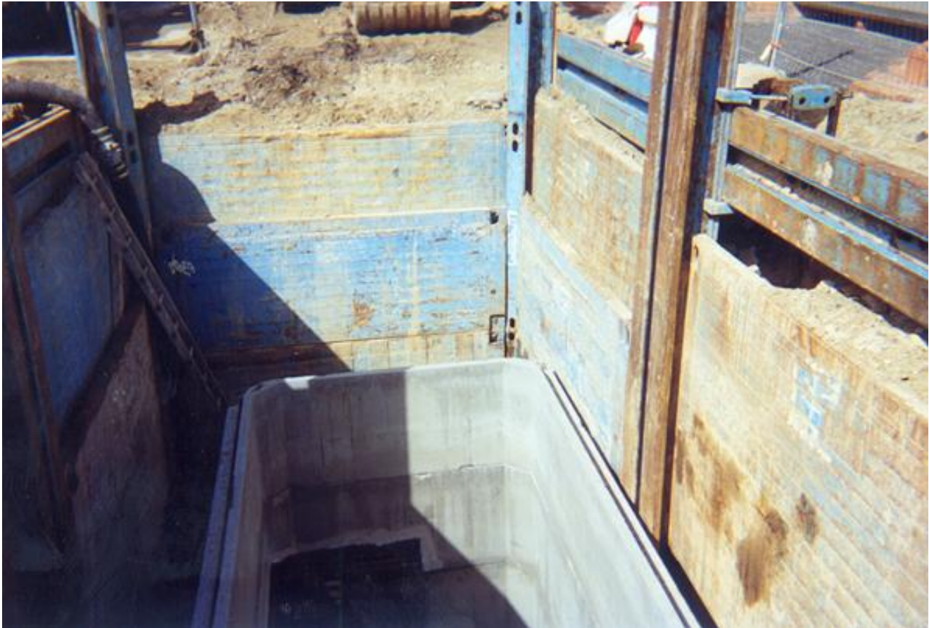
↑ Double slide rail for corner post
