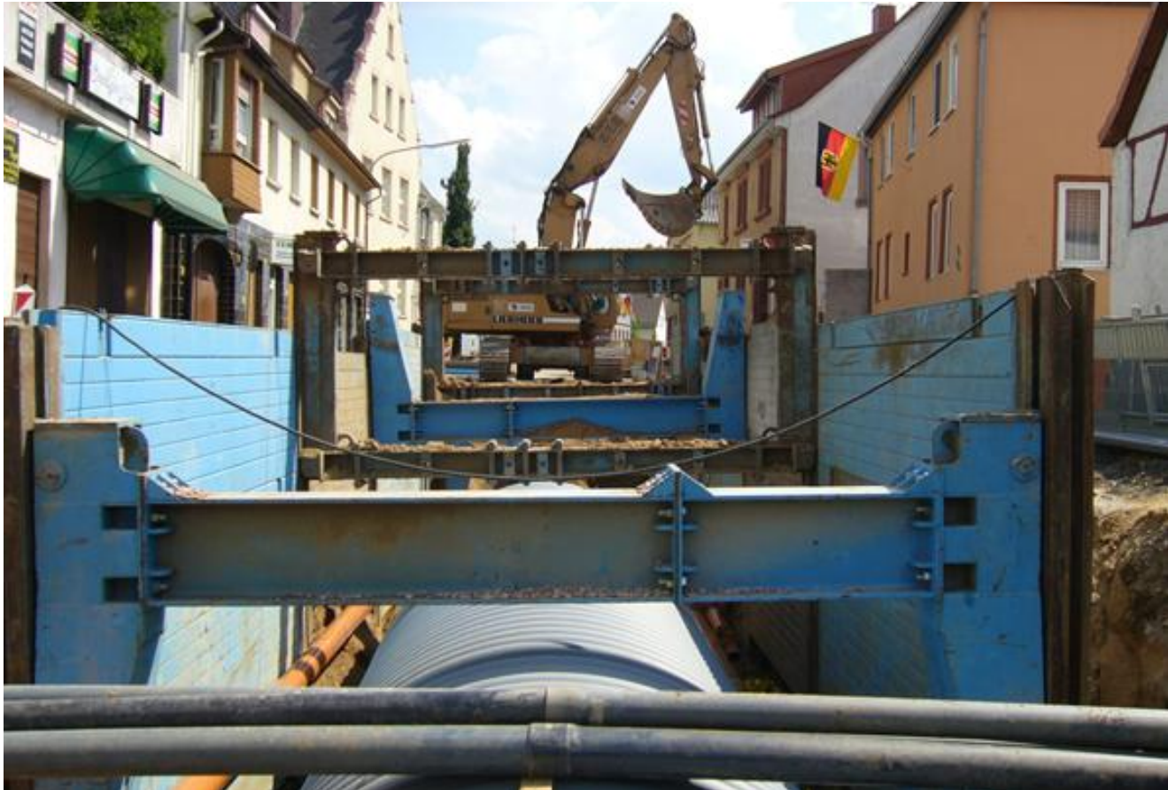
↑ Single-rail linear shoring with U-type and rectangular roller unit
